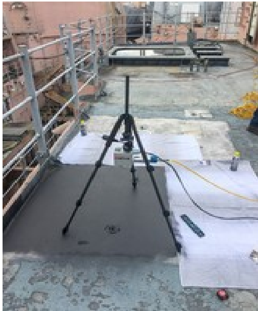
Laser Rust Removal
