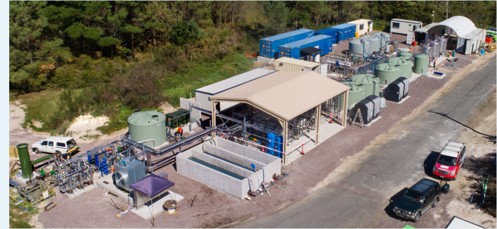
Pictured above is our 800tpd silica plant that we designed and built in 9 months; the challenge here is near-identical, but in lithium
